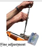
Set the insulatorbody parallel to the track by using the spirit level on the JIG.
