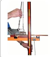
Add suspensions and control the section insulator height according to Hogging Instruction on page 1.
