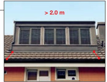
\*If a distance of 10 mm between the interception system (lightning rod) and flammable parts of the building cannot be maintained, the minimum cross section of these conductors must be  $\text{Cu } 50 \text{ mm}^2$  or  $\varnothing 8 \text{ mm}$ .
