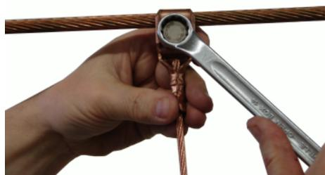
3. Install the compressed cable dropper clamp at the catenary (messenger wire) cable. Tighten the bolt with a torque wrench of 25 Nm.
